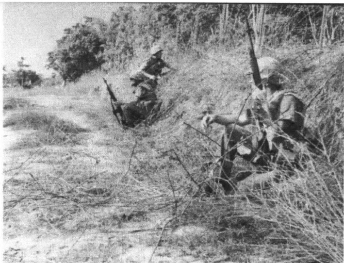
ALL IN THE JOB —Unidentified construction team hits dirt with weapons ready as Viet Cong attacks job site.
